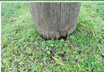
**Finding:** There is some evidence of rot in the timber. The swing frame is in generally poor condition
