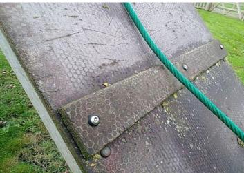
Finding: Wear on the edges of the ramp panel and treads
