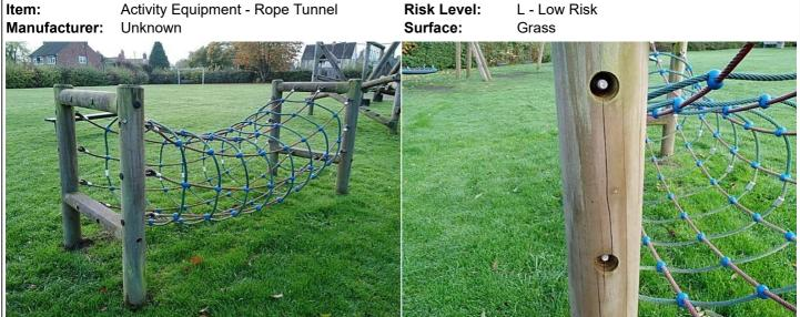
**Finding:** The timber has a number of splits/shakes or air **Action:** Monitor to ensure the splits do not cross through cracks and this may affect the stability or allow water ingress fixing points of the structure and/or cause any instability which will accelerate the rotting process
