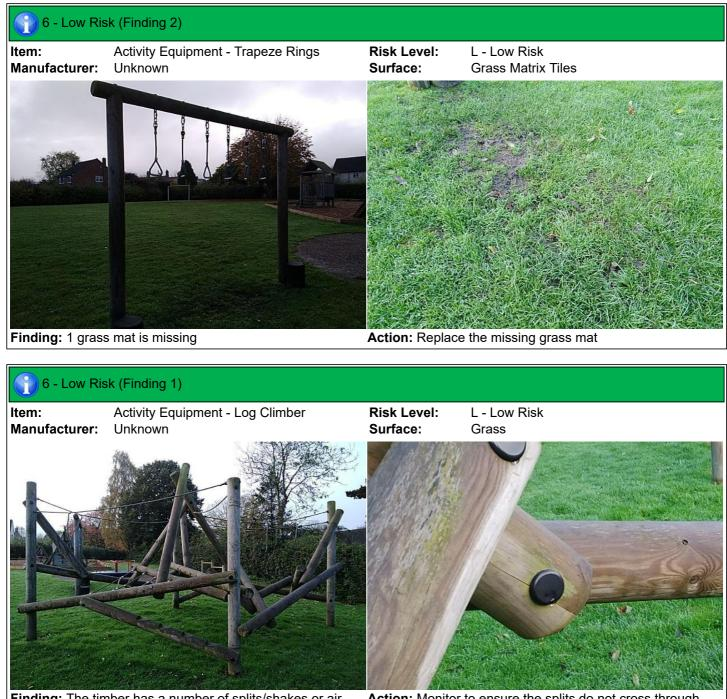
**Finding:** The timber has a number of splits/shakes or air cracks and this may affect the stability or allow water ingress fixing points of the structure and/or cause any instability which will accelerate the rotting process
