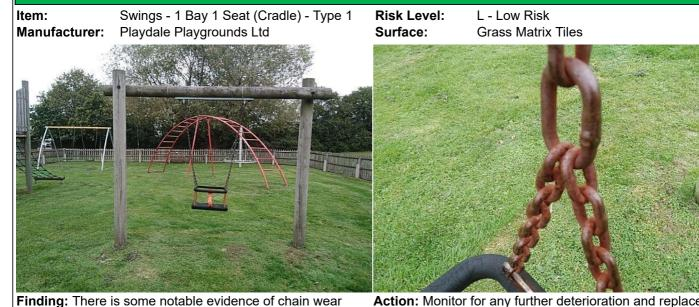
Action: Monitor for any further deterioration and replace when 40% worn
