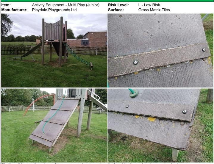
Finding: Wear on the edges of the ramp panel and treads Action: Monitor and replace as required
