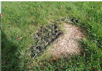
**Finding:** The edges of the grass mat surface have not been **Action:** Tuck in edges of grass mat to remove trip hazards installed in accordance with the API Code of Practice
