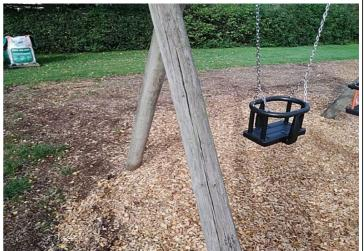
**Finding:** The timber has a number of splits/shakes or air cracks and this may affect the stability or allow water ingress fixing points of the structure and/or cause any instability. which will accelerate the rotting process. The swing frame is Consider replacing the swing frame in the longer term in generally poor condition
